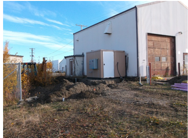
Figure 5 –Site SS019 – View of Building 1700 from the Southwest. The drywell is located to the left Building 1700
