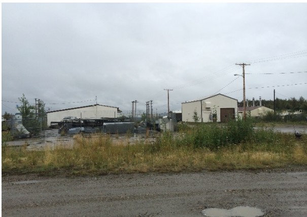
Figure 4 –Site SS006 – View of the the north side of the fenced concrete pad storage area. The building on the left is 1844 and the building on the right is 1700.
