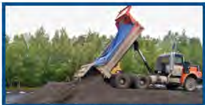
Soil remains stockpiled at the Campion air strip until the landfarm can be completed.
