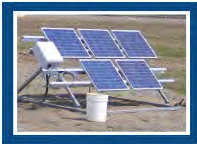
Left: Among the major things accomplished in 2010 was the installation of a bioreactor at Site SS015 just south of the runway. The bioreactor is essentially an excavation filled with locally produced mulch and vegetable oil that will break down the groundwater contaminants over time, demonstrating "green technology". The solar panels, shown here, power the pumps that recirculate the contaminated groundwater through the bioreactor.
