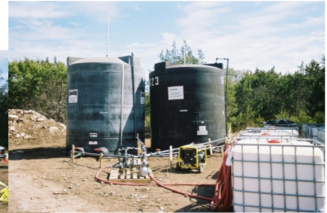
Active treatment system batch injection - Camp Bullis, 2008
