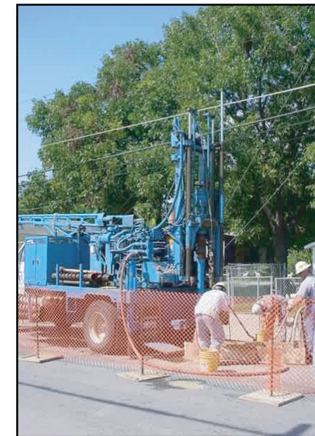
Iron filing injection method for the permeable reactive barrier on Commercial Street
