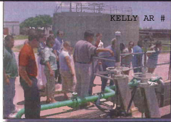
Community members tour the Groundwater Treatment Facility
