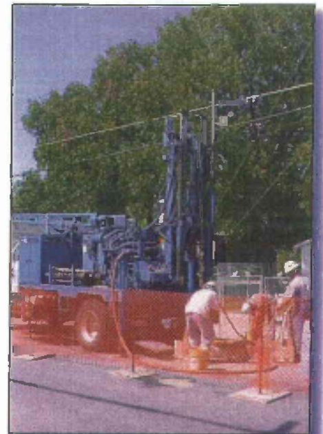
Iron filing injection method for the permeable reactive barrier on Commercial Street
