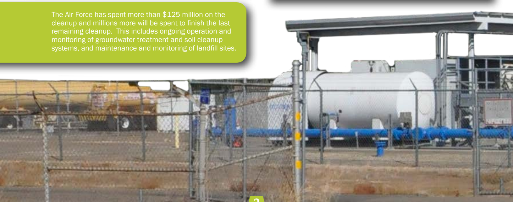
Some of the treated groundwater is discharged to surface water, while the rest is re-injected back into the groundwater. This discharge location is near the SAC/Main Base treatment plant located on the northwest corner of Mather.
