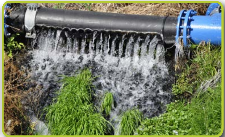
Some of the treated groundwater is discharged to surface water, while the rest is re-injected back into the groundwater. This discharge location is near the SAC/Main Base treatment plant located on the northwest corner of Mather.
