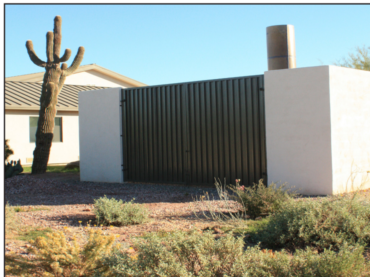
Part of the ST035 SVE system operates within a block wall treatment building on the ASU Polytechnic Campus.
