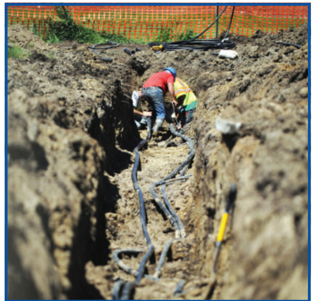
Geothermal Project at Minot AFB, North Dakota
