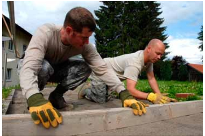
Staff Sgt. Zach Whitener, 184th Communications Flight, and Tech. Sgt. Karey Haukom, 184th Civil Engineer Squadron, resurface a walkway at the NATO school on base.
