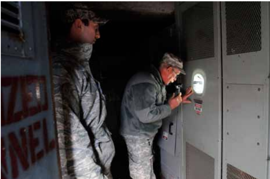
SrA Jared Brotsky, of the West Virginia ANG’s 130th CES, and Sgt. 1st Class Marty Newman, 3664th Maintenance Co., WVNG inspect the electrical components for a boiler in the basement of an apartment complex in Queens, N.Y.
