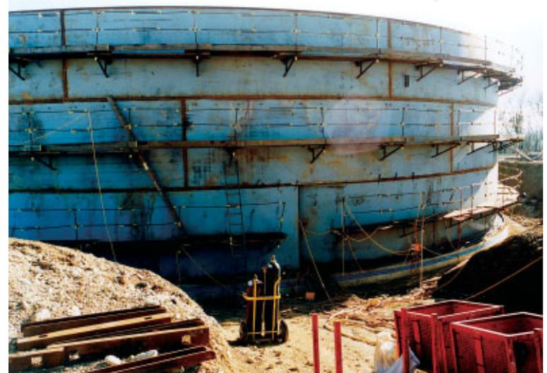
**Above right: Preparing reinforcement cage for 2,500-cubic-meter tank base. Below right: Welding steel sections of 5,000-cubic-meter tank. (photos by Philip Lane Company, Orpington, Kent, United Kingdom)**
