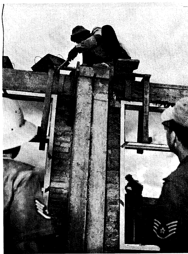
Viet Nameese workers complete the brick understructure of a masonry barracks as AF personnel supervise.
