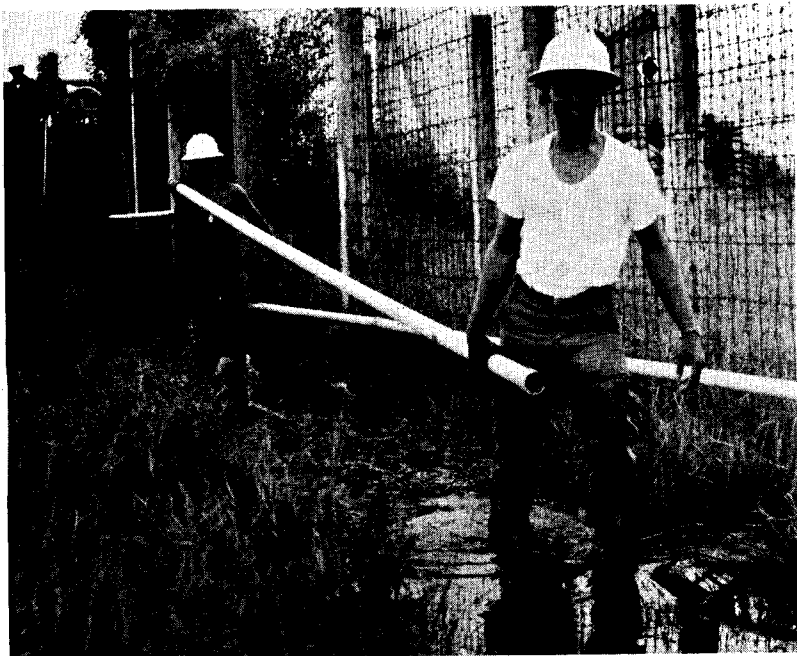
Pipe-laying operation at Tan Son Nhut.
