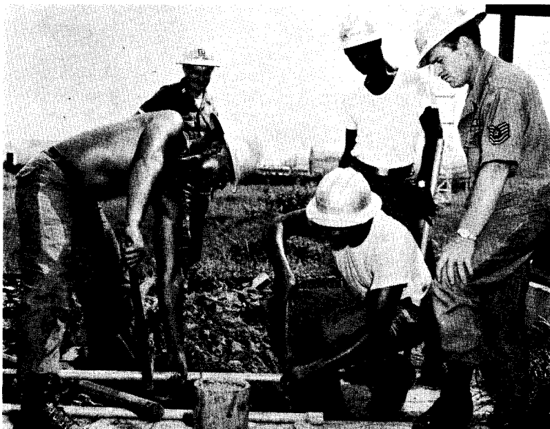
MAC plumbing team had problems threading foreign pipe.
