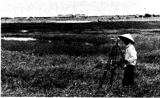
Bien Hoa—A Vietnamese surveyor checks dimensions for what will soon be a jet parking apron for F-100 Supersabres.
