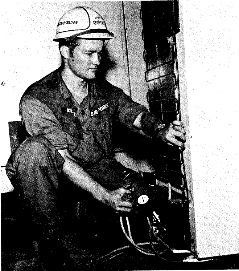
REFRIGERATION: Airman 2/c Paul Kessler, a refrigeration specialist tests a cooler at the Pleiku Air Base.
