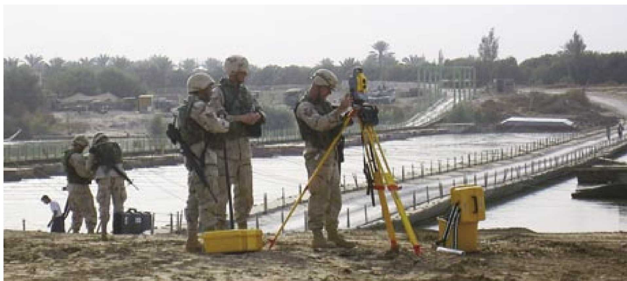
Members of the 240th CEF joined Active Duty engineering assistants to help the U.S. Army build bridges in Iraq. These two float bridges give civilians and coalition forces an important river crossing. (photo by Maj Phil Landeros)
