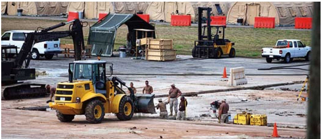
“Dirt Boys” from the 474th ECES prepare to lay a permanent foundation for Naval Station Guantanamo Bay’s new military commissions courtroom. (photo by Army Sgt. Sarah Stannard)
