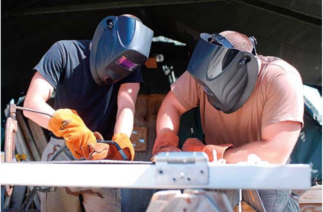
SrA Nick Skinner and SSgt John Heiser weld a detainee cell door at Naval Station Guantanamo Bay. Both are members of the 474th ECES, which was assigned the task of building the Expeditionary Legal Complex. (photo by Army Spc. Shanita K. Simmons)
