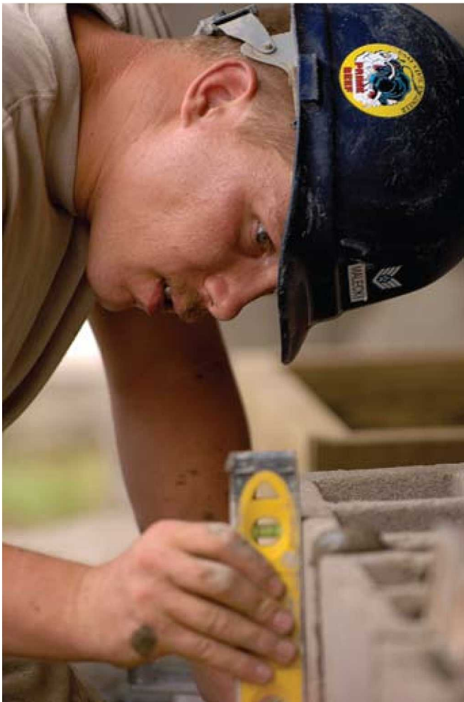
SSgt Arthur Malecki of the 5 CES, Minot, N.D., helps make repairs to The Best Hospital in West Demarara, Guyana. (U.S. Navy photo by MC Ernest Scott)
