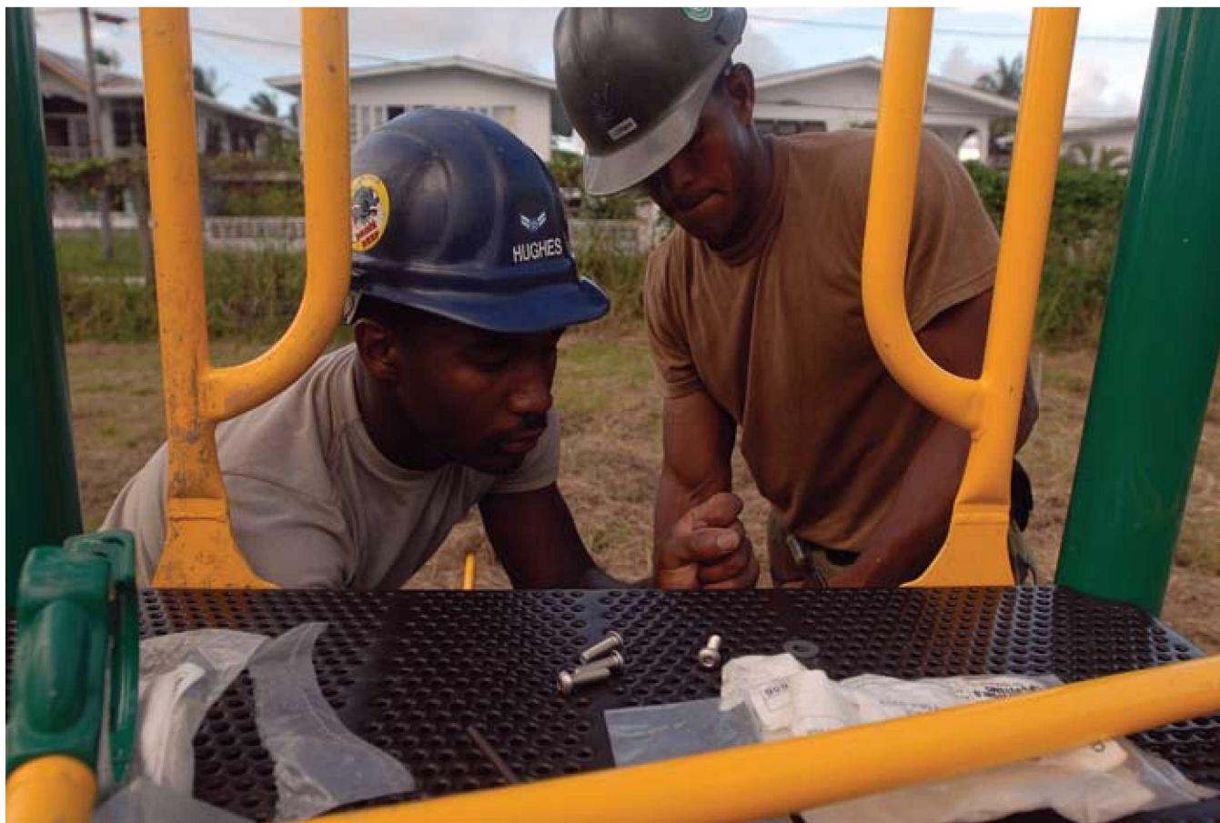
A1C Pasha Hughes, left, of the 5 CES, and Navy Seabee Hugo Lerma work together building a new playground for a local community in Guyana. (U.S. Navy photo by MC2 Gina Wollman)
