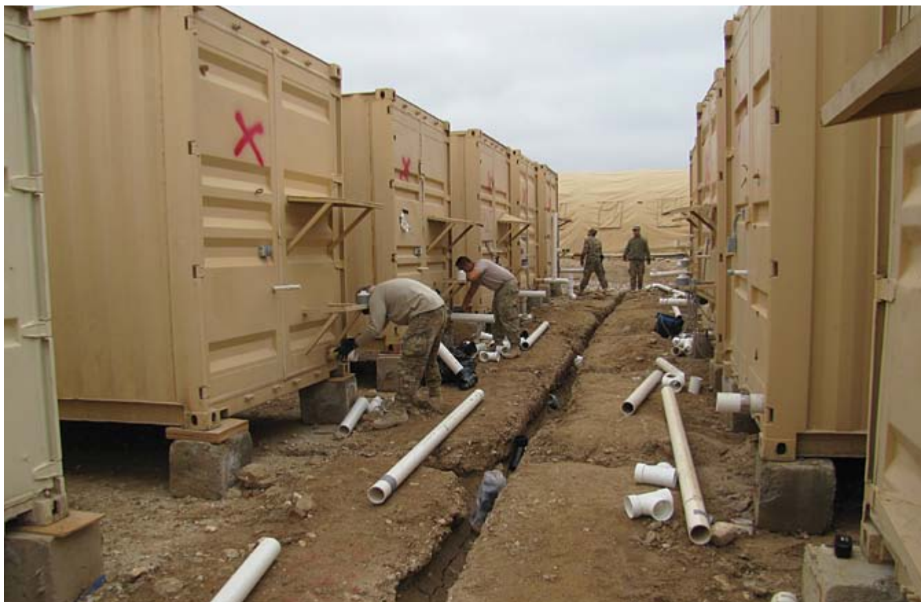
(facing page) Dirt Boyz from the 577 EPBS pour the first lane of the wash rack for a retrosort yard at Camp John Pratt, at an undisclosed location in Southwest Asia. (above) Water and fuels system maintenance craftsmen from the 577 EPBS dry fit sewage lines for latrine and shower units at a life support area at Camp John Pratt. (U.S. Air Force photos)
