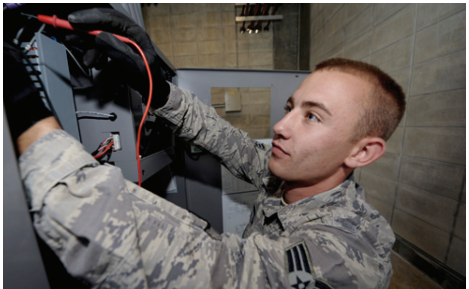
SrA Derek Hunter checks electrical circuits on an HVAC system at Kadena Air Base, Japan. Base officials replaced old, outdoor AC chillers with protected, indoor equipment to save the Air Force potentially millions of dollars in parts and energy. (Photo by SSgt. Jonathan Steffen)
