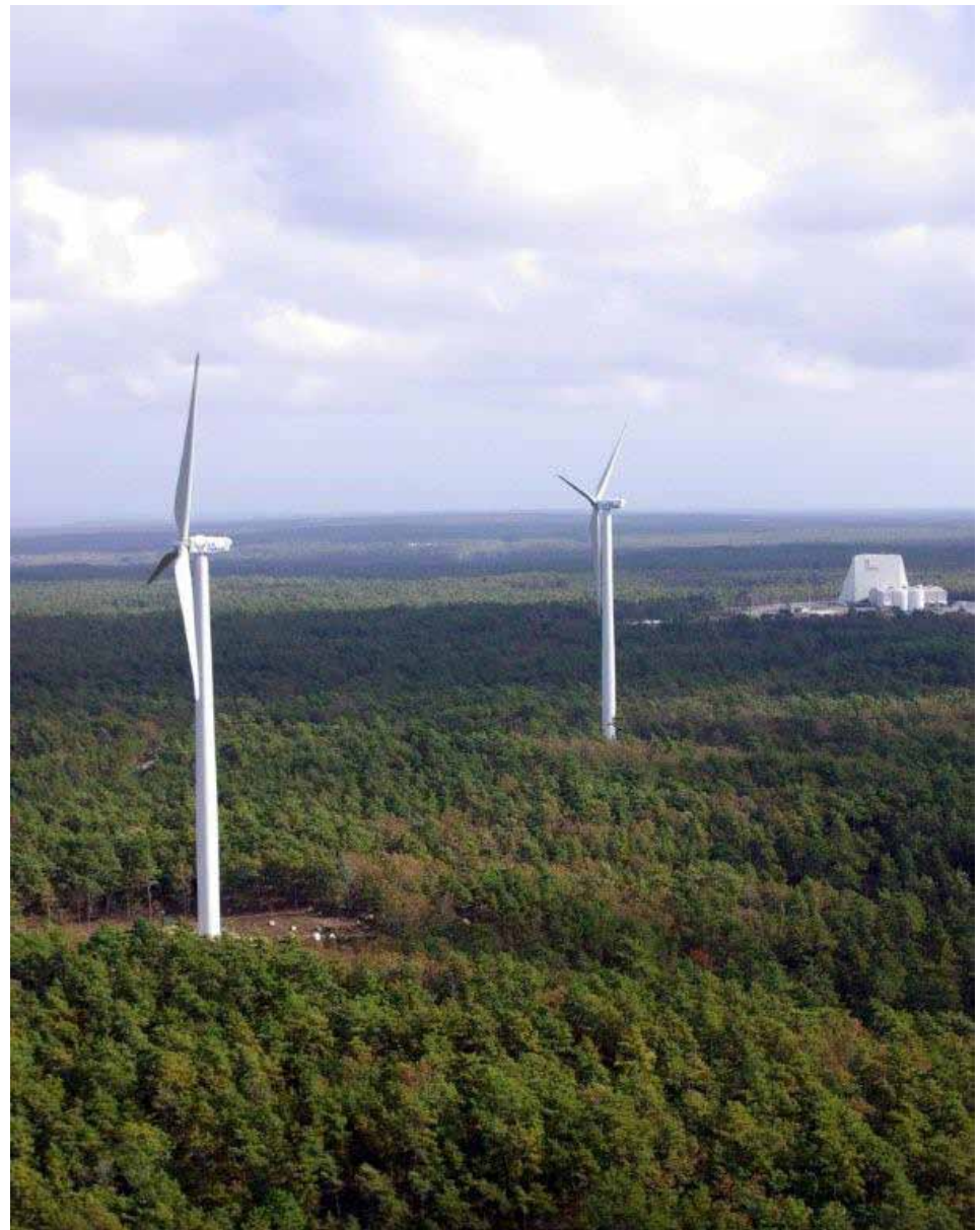
Air Force Space Command is preparing to install two 1.6 megawatt utility-scale wind turbines at the Cape Cod Air Force Station, Mass., located at the Massachusetts Military Reservation. The new turbines will be similar to these two already in place at the MMR and will offset over 50 percent of the station's annual electrical purchases. (U.S. Air Force photo)
