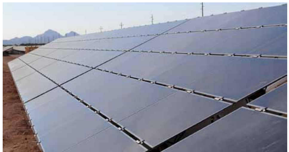
The new 14.5-megawatt photovoltaic solar array at Davis-Monthan Air Force Base, Ariz. will join other solar projects at the base already in place for base housing. Completion of the project is expected by December 2012 and will provide 35 percent of the base's power needs. (U.S. Air Force Photo /Staff Sgt Jacqueline Romero)
