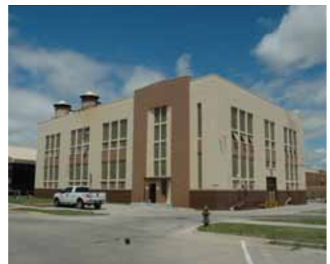
This is one of three central heat plants at Tinker AFB, Okla., scheduled to be decentralized. The plant produces steam which is piped throughout the base for heating and other processes. (U.S. Air Force photo/Mr. Bill Dalky)
