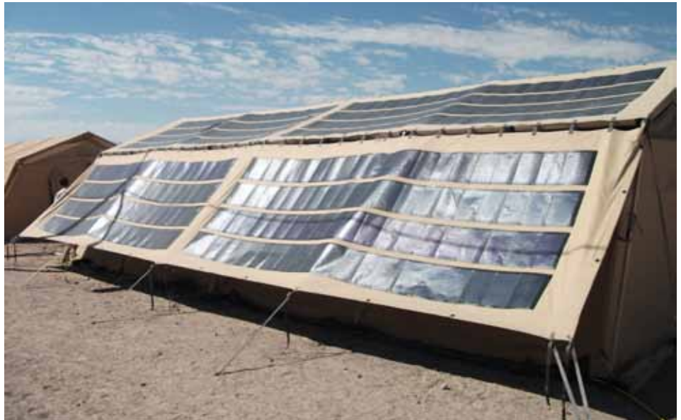
A shade fly with photovoltaic panels for generating power is just one of the energy saving technologies being tested and implemented in the new program, "Advanced, Energy Efficient Shelter Systems for Contingency Basing and Other Applications". (Photo by Mr. Rod Fisher)
