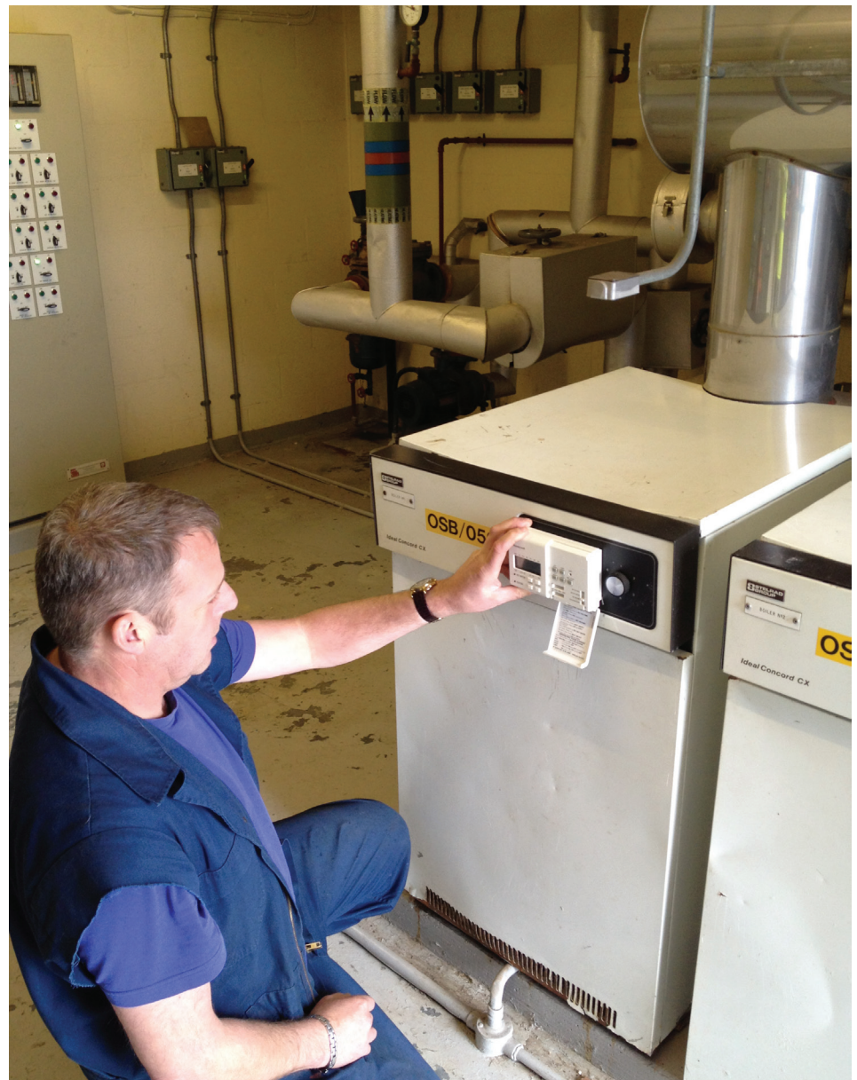
RAF Alconbury HVAC Foreman, Mr. Stuart Chalmers, installs a low-cost mechanical time clock on a boiler. This small device is expected to save 35 percent of the fuel used by the boilers every year. (Photo by Mr. Sam Williams)
