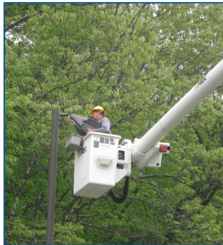
A contractor installs a new light emitting diode street fixture at New Boston Air Force Station, N.H. It is one of 15 Air Force Space Command installations to receive the energy-saving lights. AFSPC centrally purchased 6,600 lights which will save $975,000 annually on reduced operations and maintenance costs. (U.S. Air Force photo)
