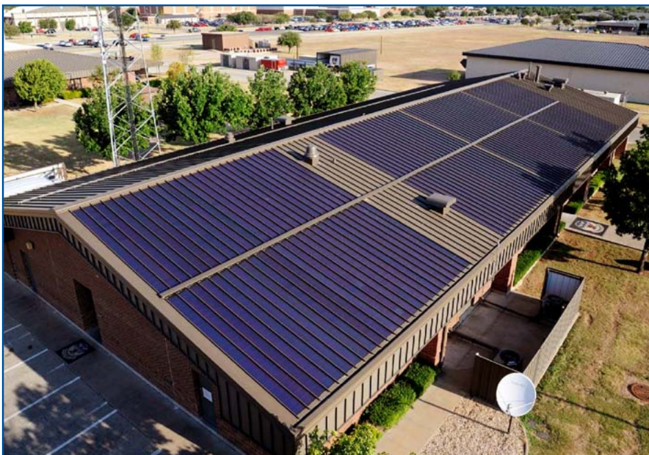
GOODFELLOW AIR FORCE BASE, Texas -- A one of its kind roof here is attracting national attention. Six sustainable technologies installed atop the base's security forces building reduces the utility bill, produces energy and captures rainwater for irrigation. (U.S. Air Force photo/Eddie Green)
