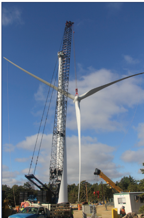
The turbine's blade assembly is hoisted into place atop the 260-foot tall tower. (U.S. Air Force photo)
