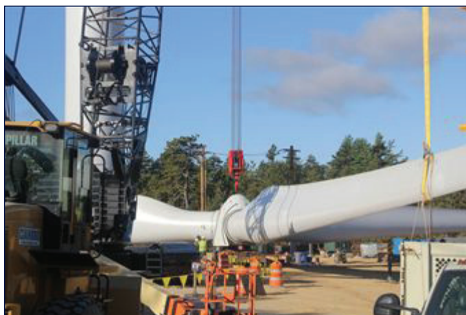
The turbine's blade assembly is hoisted into place atop the 260-foot tall tower. (U.S. Air Force photo)
