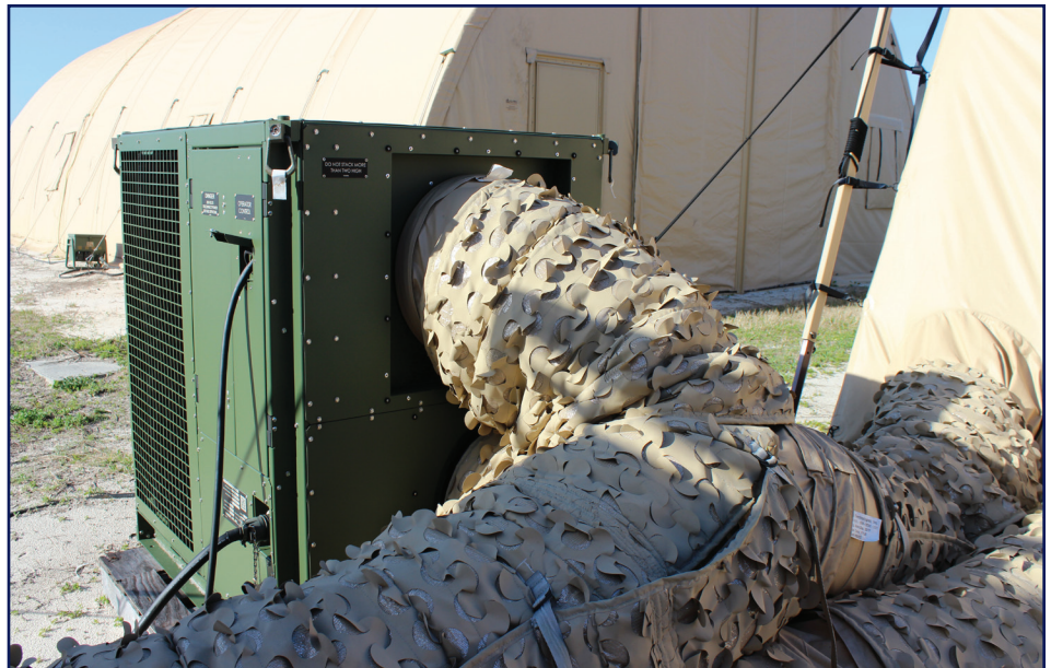
New energy-efficient environmental control units like this one with thermal coating and insulated ducts along with other initiatives helped the Air Force cut its expeditionary facility energy use by more than 60 percent in recent tests. (U.S. Air Force photo/Jennifer McCabe)
