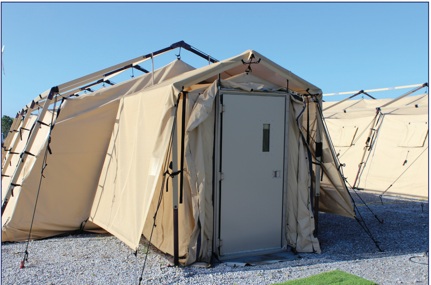
This shelter with a vestibule, hard door and shade fly is similar to those tested in Southwest Asia. These energy-saving measures along with photovoltaic flies, insulated liners, LED lights, thermal coatings and improvements to environmental control units reduced energy use 63 percent in recent tests. This shelter is on display at Tyndall AFB, Fla. (U.S. Air Force photo/Jennifer McCabe)
