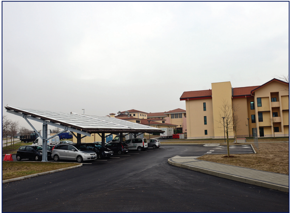
Solar water-heating panels for the dormitories on Aviano Air Base, Italy, are comprised of 64 panels. This renewable energy initiative provides 10,000 liters of hot water production capacity, and saves approximately $4,000 a year. (U.S. Air Force photo/Senior Airman Matthew Lotz)
