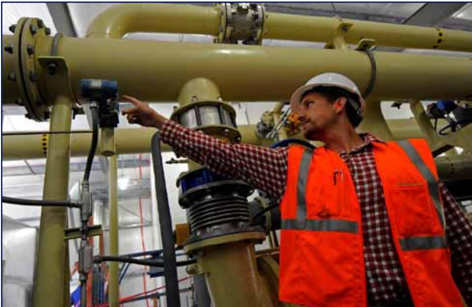
Greg Mitchell checks the pressure on the landfill gas processing module at the Anchorage Landfill in Alaska. The module cleans and dries landfill gas before it is sent to the Joint Base Elmendorf-Richardson landfill gas waste-to-energy plant. The project is one of eight Air Force projects selected as 2014 Federal Energy Management Program award winners. (U.S. Air Force photo/Tech. Sgt. Brian Ferguson/Released)
