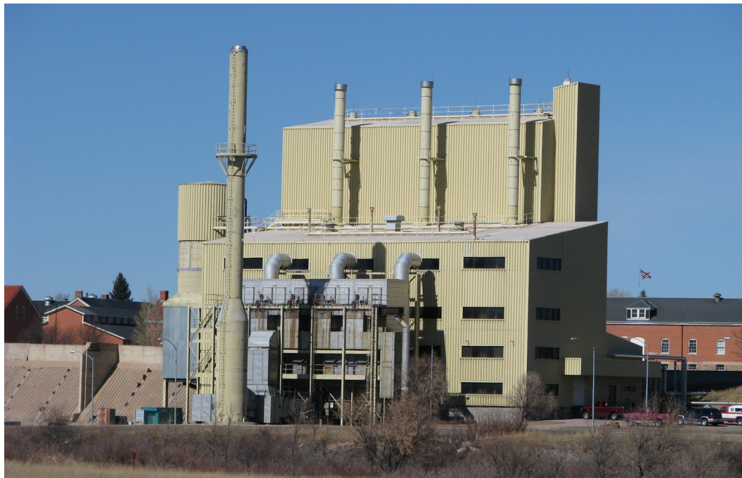
The central heat plant at F.E. Warren Air Force Base, Wyoming, built in 1981, was suffering more than 50-percent energy losses due to age and deteriorating distribution lines. The base used the Energy Conservation Investment Program to fund the decentralization project that included fitting 85 base facilities with their own natural gas boiler, saving $740,000 per year in energy costs. (U.S. Air Force photo Released)
