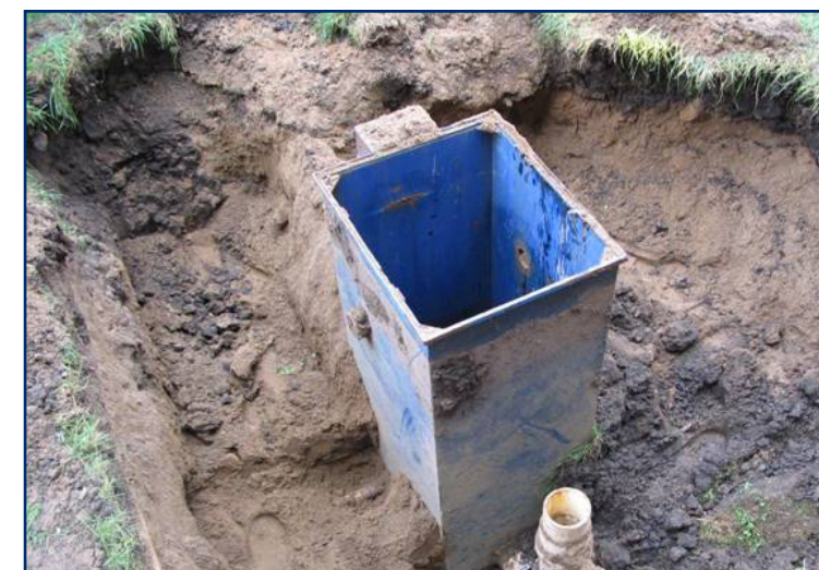
The oil/water separator removed near Building 933.
