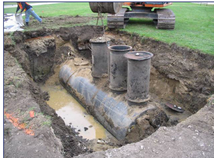
The oil/water separator removed near Building 711.
