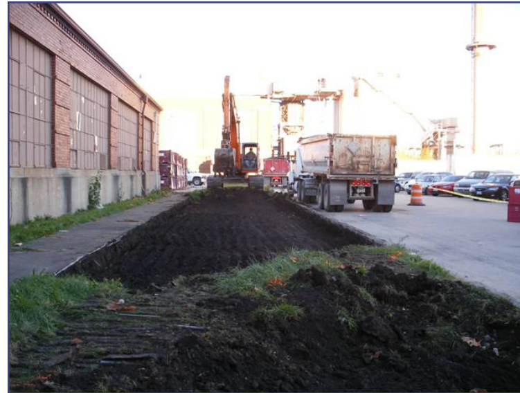
Contractors remove soil near Building 1.
