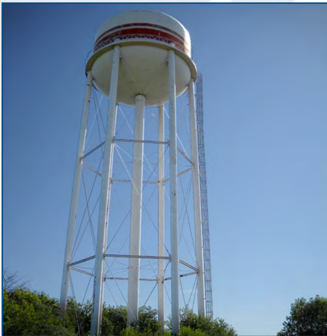
Water Tower Facility 968 is one of six "Group 1" sites closed and now available for transfer and redevelopment.
