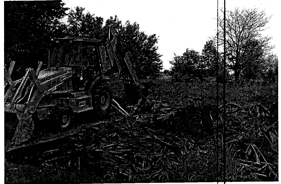
Sampling of Salt Fork Creek Dredge Piles
