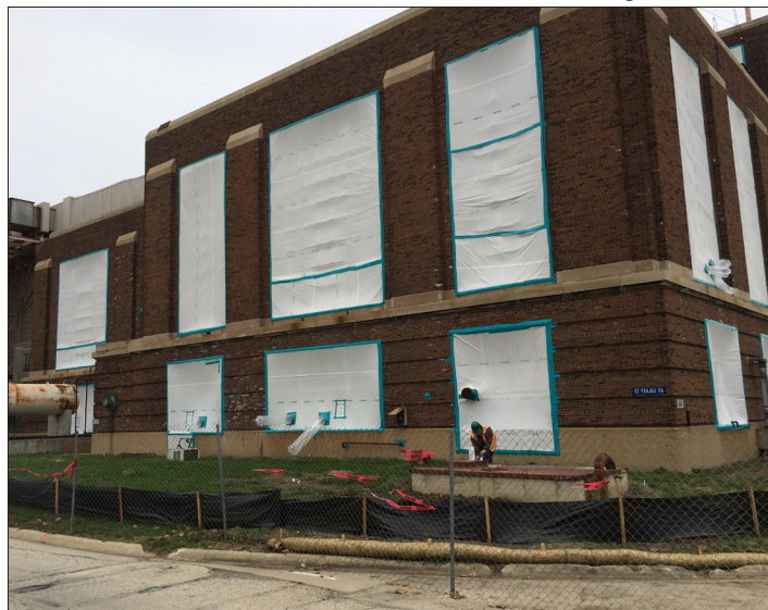
Sealant over the steam plant's openings bows inward as the vacuum system inside applies negative pressure, preventing the escape of asbestos into the surrounding area.
