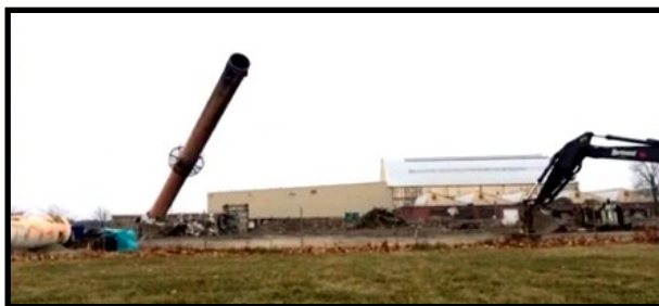
Photo of the smoke stack at the Chanute steam plant as it is being demolished via a "controlled-tilt" method. Photo courtesy: North Wind Services
