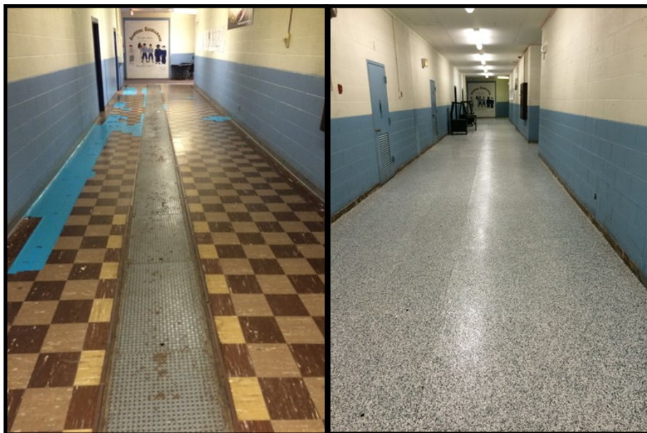
Typical hallway in Bldg. 12—Lincoln's Challenge Academy showing condition of ACM floor tile before ACM abatement and after abatement. Photo Courtesy, AF contractor, CB&I
