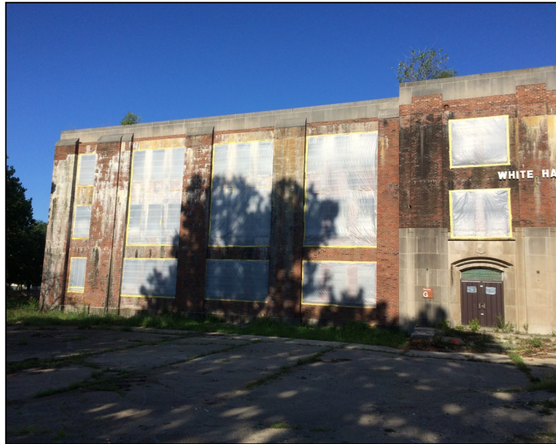
White Hall windows sealed prior to abatement. Photo Courtesy, AF contractor, CB&I
