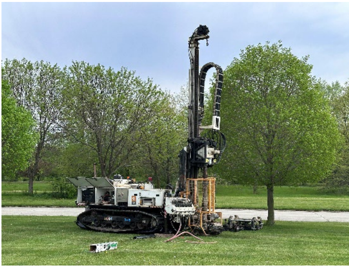
Figure 1: Monitoring Well Boring
