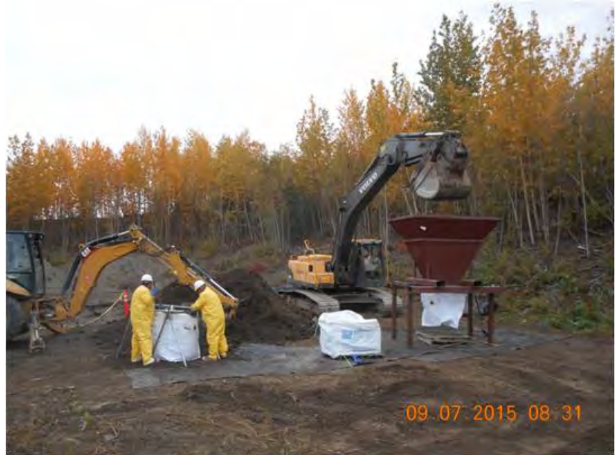
Placing contaminated soil in super sacks for off-site disposal
