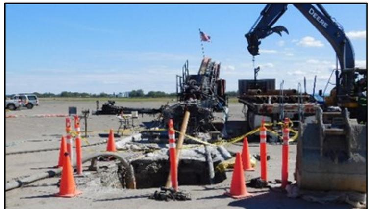
AF contractors conduct horizontal well drilling at the former Galena FOL. Photo Courtesy: AF Contractor
