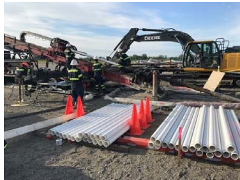
Horizontal well installation in 2017
