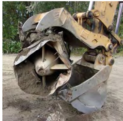
Site DP023 2019 Excavation
