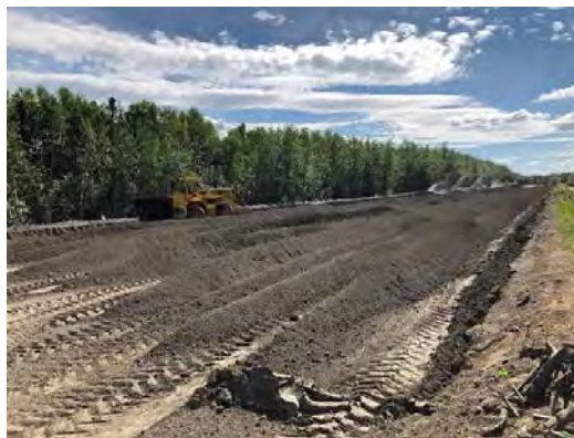
Tilling Operations at the Landfarm
