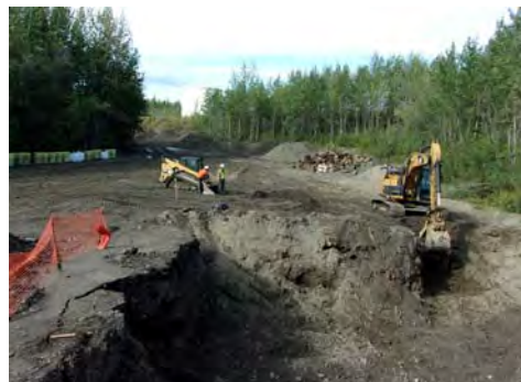
2019 Excavation at Disposal Site West of Dike (Site DP023)
