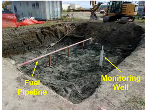
Site SS018 Excavation Area
