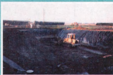
Backfilling of Excavation Pits 7080 and 7090
