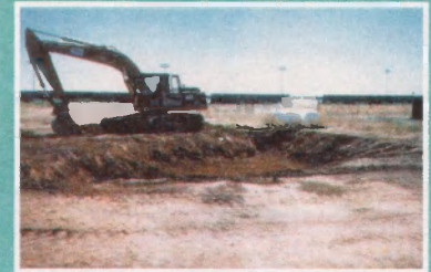
Excavation of Refuse Pits
