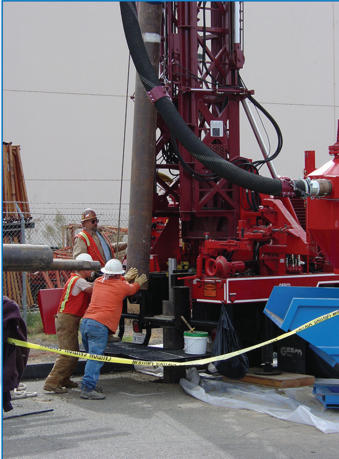
Workers install one of the 103 groundwater extraction wells at McClellan. The McClellan groundwater treatment system is successfully keeping the problem in check.
