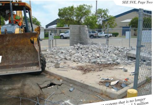
Crews dismantle an SVE treatment systems that is no longer needed near the former Building 1048. More than 1.5 million pounds of contaminants have been removed through soil vapor extraction at McClellan.
