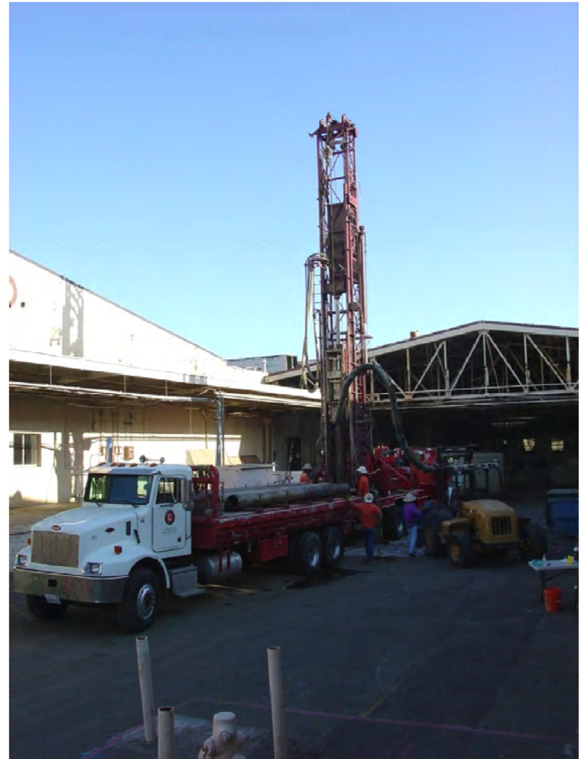
Drilling new extraction well
