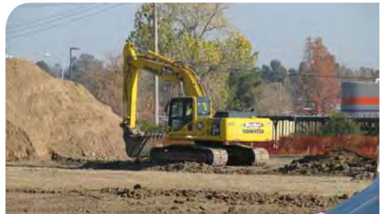
The Air Force removed some 9,500 cubic yards of contaminated soil from the former skeet range in the northwest portion of the former base and disposed of it in a licensed landfill.
