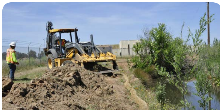
Excavation of tailings piles at Magpie Creek.
