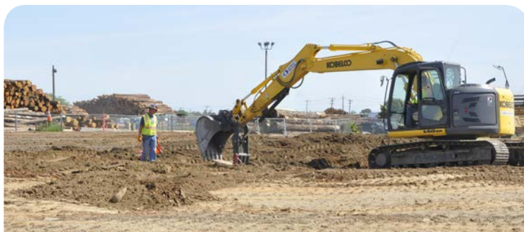
Excavation at CS 24
