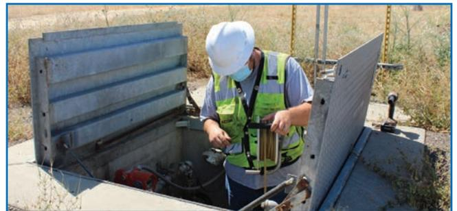
Air Force Civil Engineer Center environmental contractor, Aaron Johnson, AECOM Field Technician, inspects a groundwater extraction well at the former McClellan Air Force Base. Extracted groundwater is processed at a nearby treatment plant where clean groundwater is then returned to local creeks.
