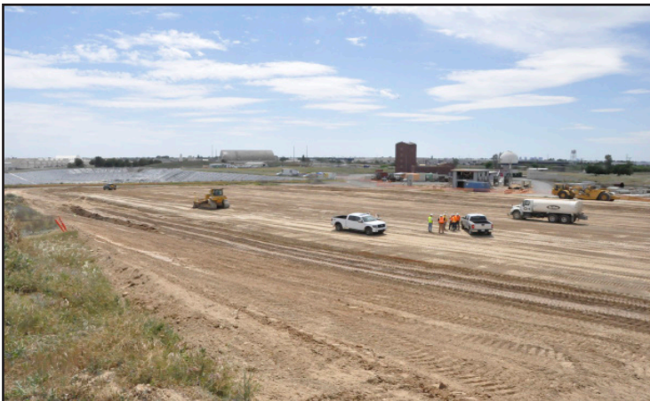
A consolidated cap was constructed on PRL008 in 2015.
