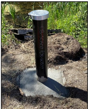
Left: A completed stick-up well.
