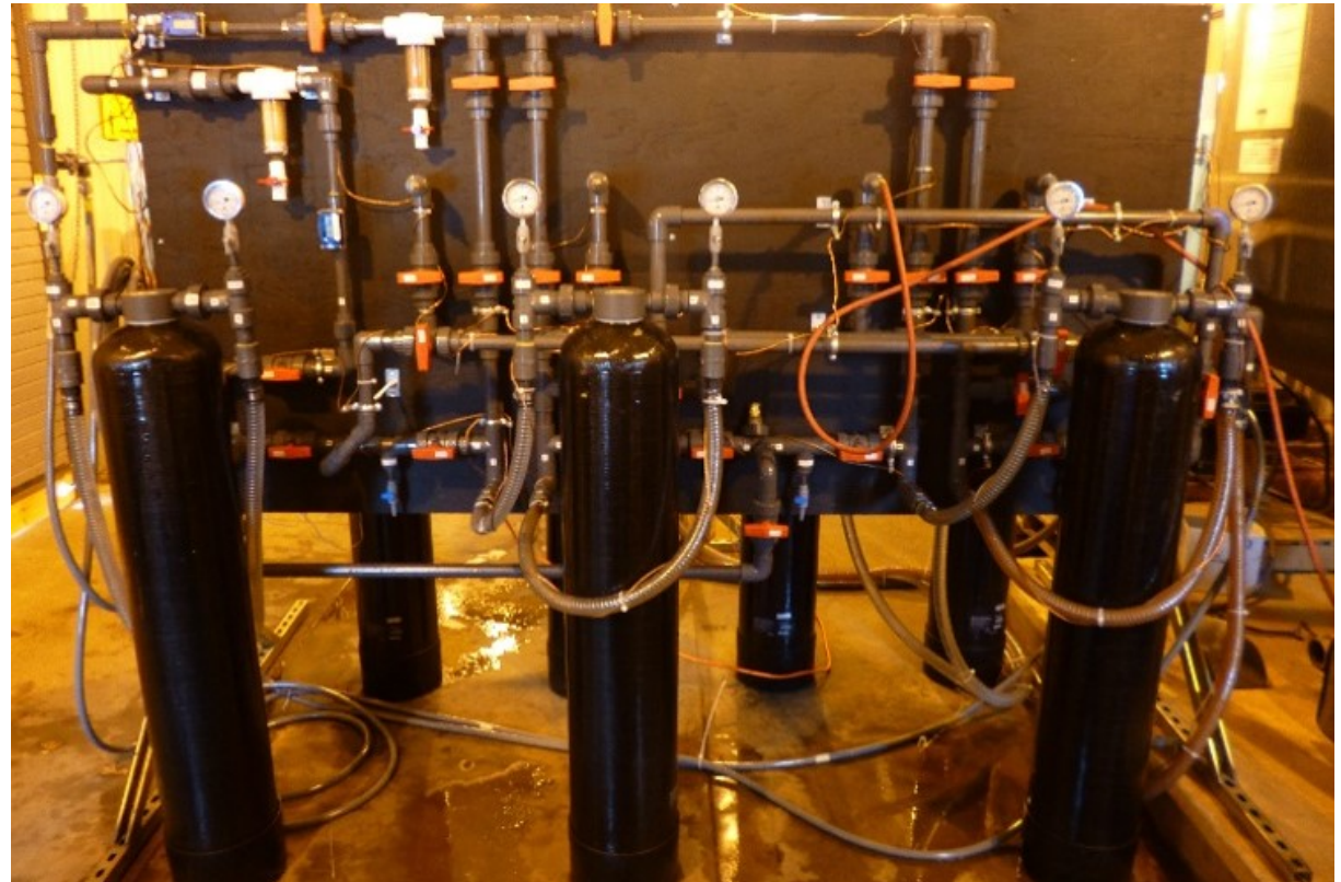
Pilot Scale Testing (at the Fire Training Area)
