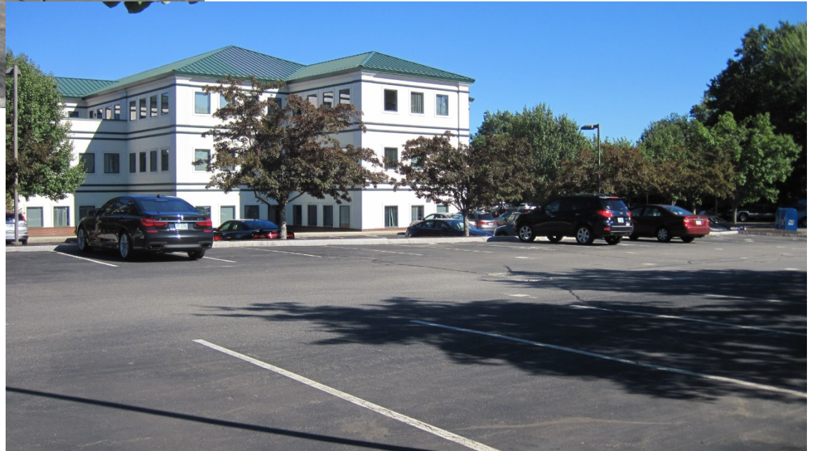
Site after injections complete
